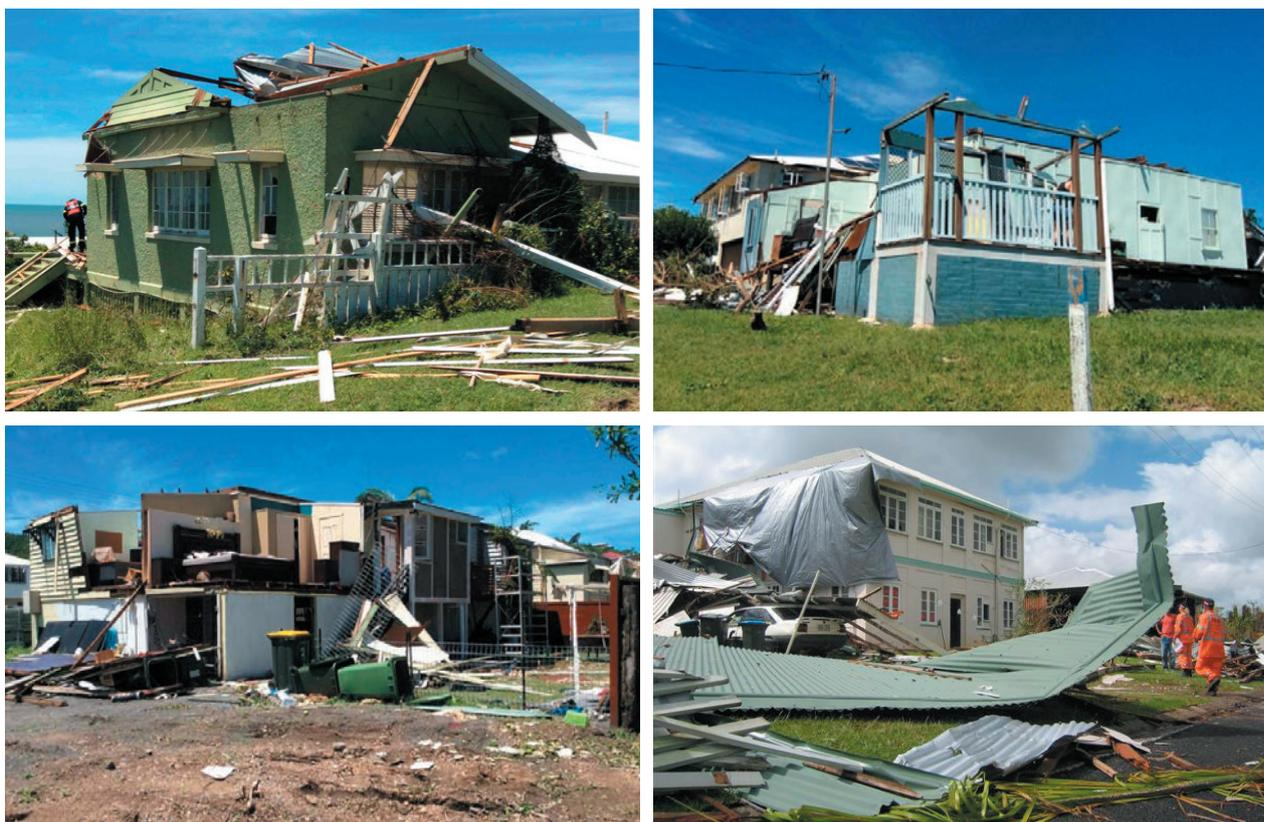
Figure 8: Damage to buildings in Yeppoon in the aftermath of Severe TC Marcia, 2015. Source: Queensland Fire and Emergency Services
