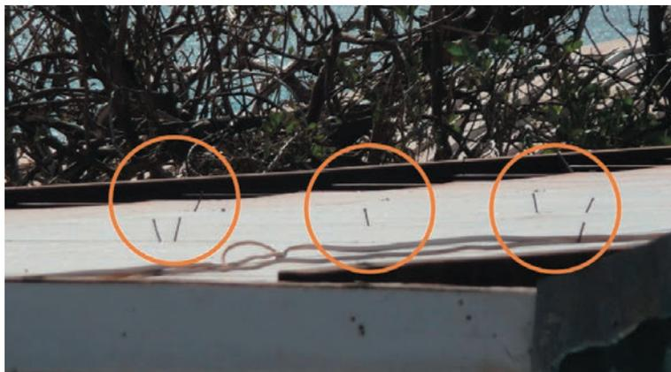
Figure 15: Loose fixings resulting from a previous cyclone.
