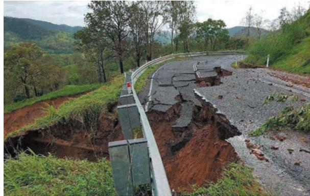
Figure 26: Serious damage around Sarina Range due to landslips from Severe TC Debbie. Source: Loretta MacGregor
