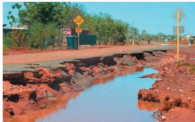
Figure 10: Scour damage to a road from storm surge.
