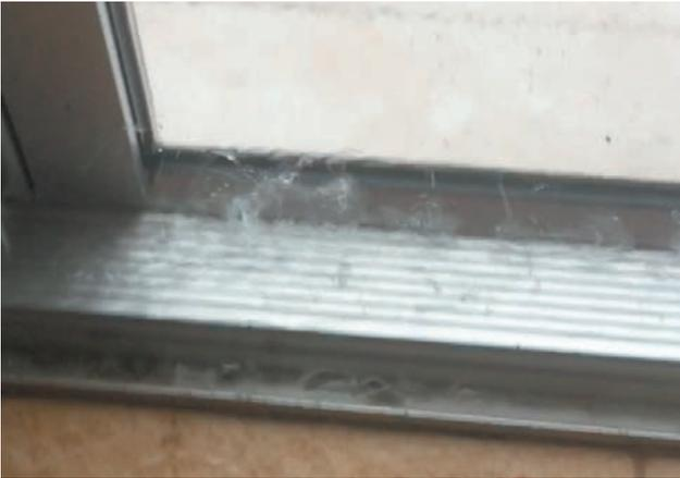
Rainwater bubbling through weep holes in windows.
