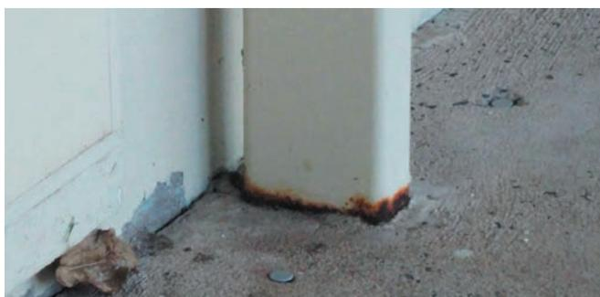
Figure 12: Signs of rust at the bottom of a verandah post.
