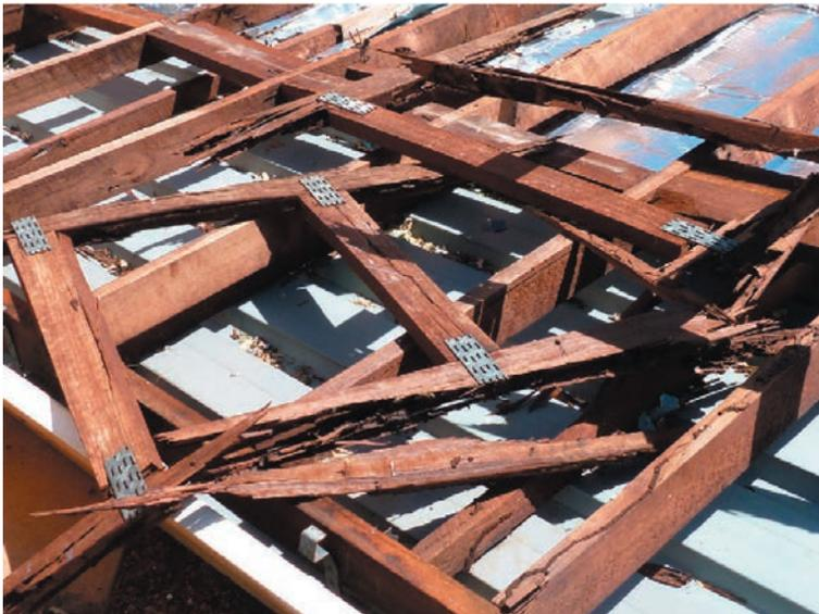
Figure 14: Termite damage to roof timbers.
