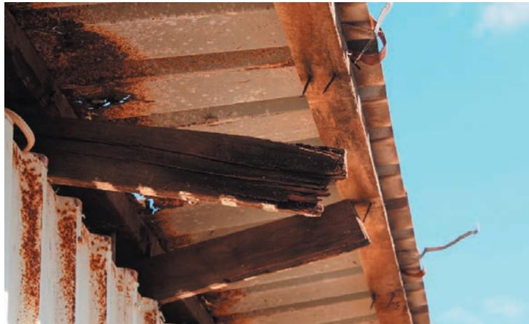
Figure 13: Timber rot in a rafter.
