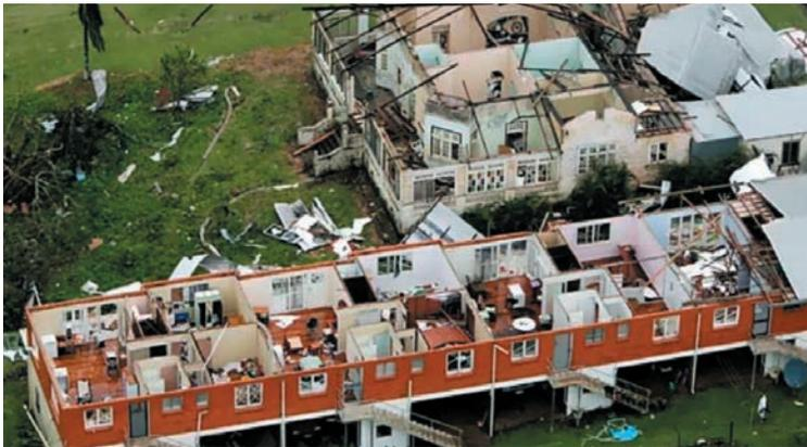
Figure 21: Houses and apartment blocks with their roofs blown off in Innisfail after Severe TC Larry struck in March 2006. Source: Mark Baker(AP)
